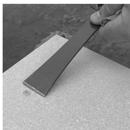
Remove protective glue-dot spacers with a sharp edge. Clean any residue or excess bonding material with solvent based cleaner.
