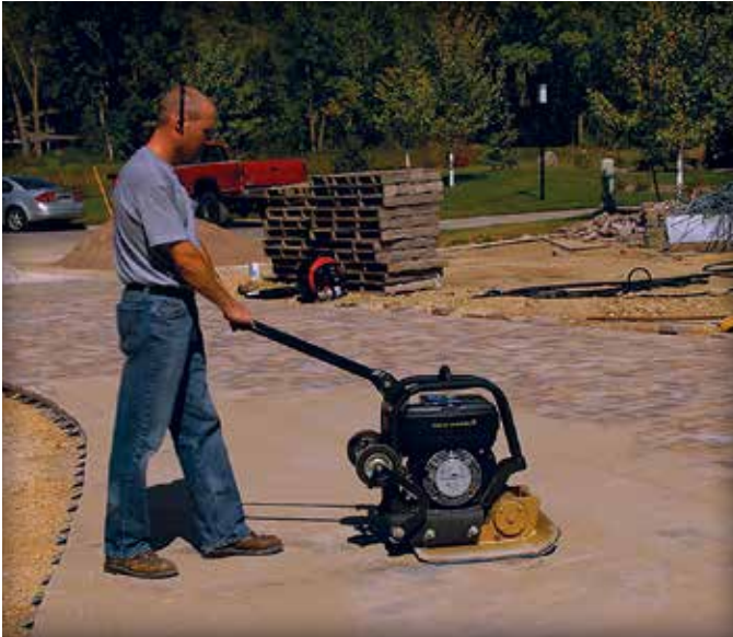
Figure 11. Vibrating sand into the joints.
