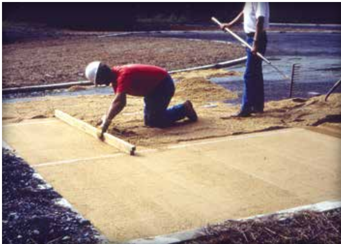
Figure 6a & 6b. Screeding the bedding sand.
