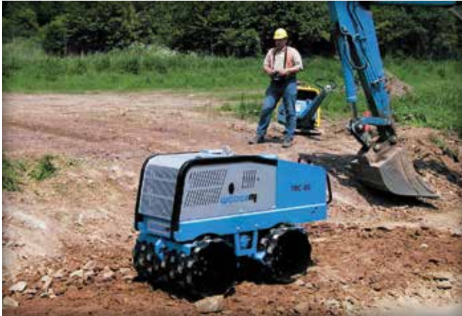
Figure 2. Compacting the soil subgrade.
