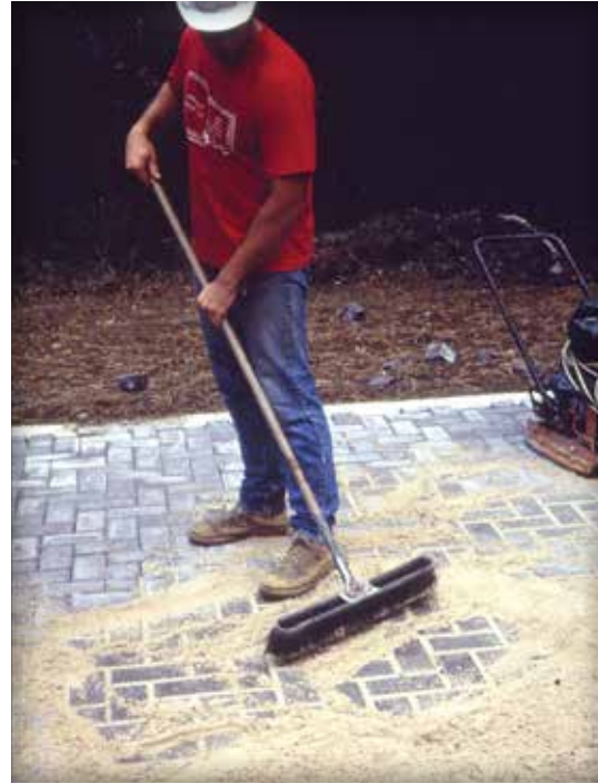
Figure 10. Spreading the joint sand.
