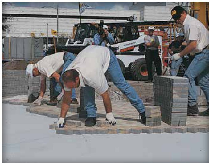
Figure 7. Placing the concrete pavers.
