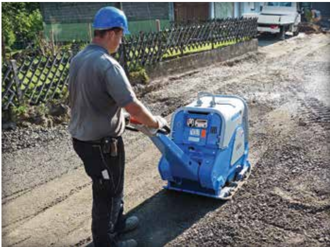
Figure 4. Base compaction with a reversible plate compactor.
