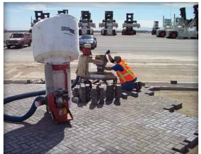
Figure 8. Saw cutting pavers.
