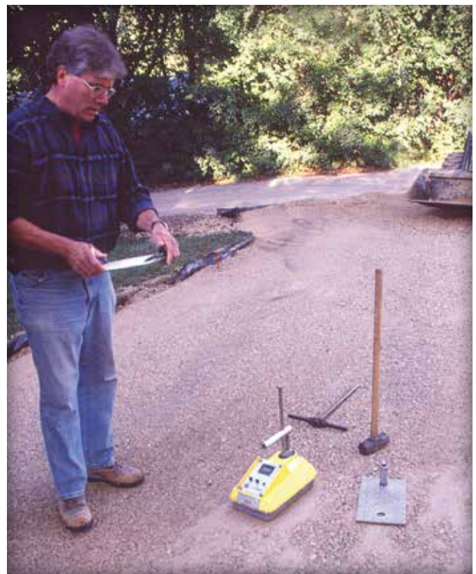
Figure 5. Density testing of the aggregate base with a nuclear density gauge.
