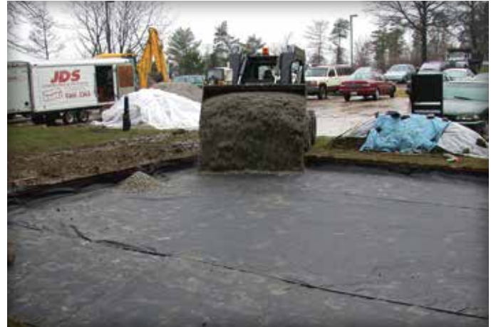
Figure 3. Application of the geotextile under aggregate base.
