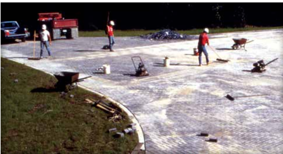
Figure 12. Removing excess sand from the finished surface will make the pavement ready for traffic.
