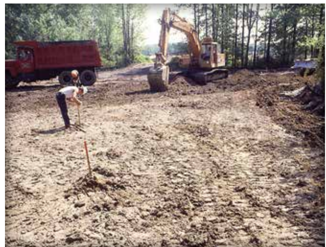
Figure 1. Excavation of the soil subgrade and placing grade stakes.
