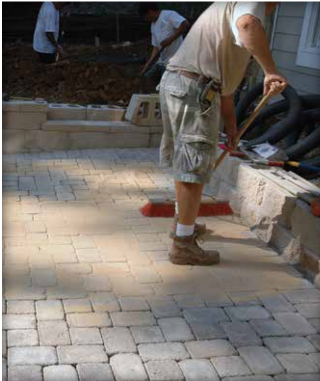
Figure 8. Spreading joint sand over the installed concrete pavers.
