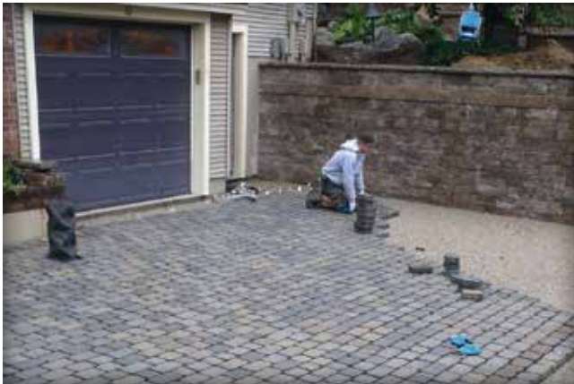
Figure 11. Concrete pavers installed to accommodate permeable bedding and jointing materials, all supported by a permeable stone base.
