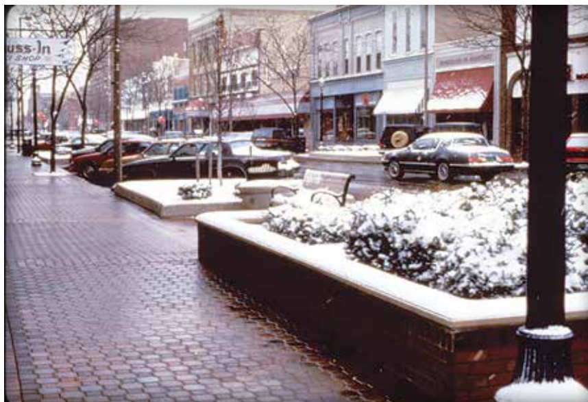
Figure 1. A snow melting system under concrete pavers in downtown Holland, Michigan has performed well since 1988.
