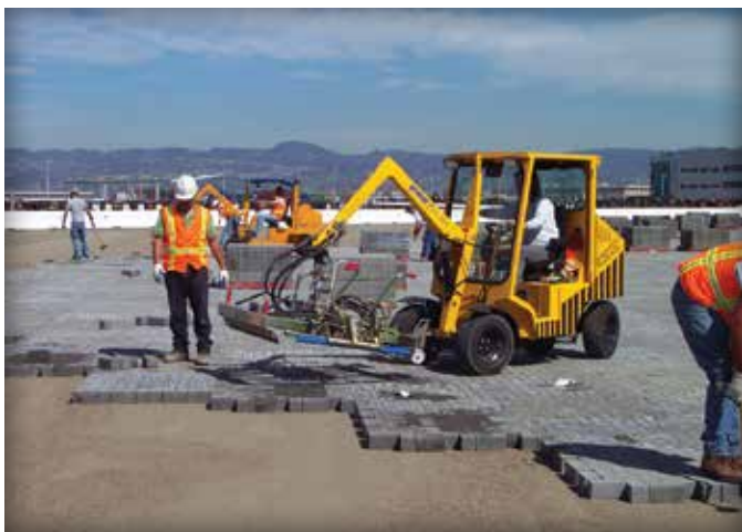
Figure 5. Motorized equipment with a hydraulic clamp.
