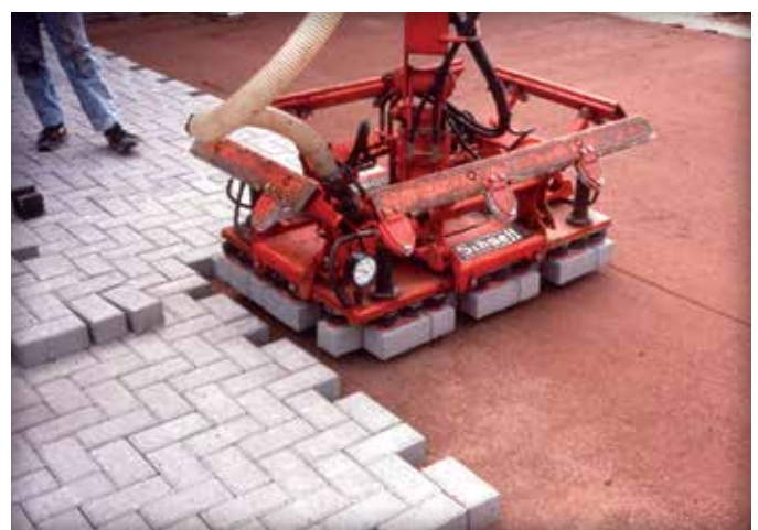
Figure 6. The vacuum head over the paver layer.
