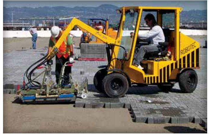
Figure 4. Hydraulic clamp picking up layer of pavers
