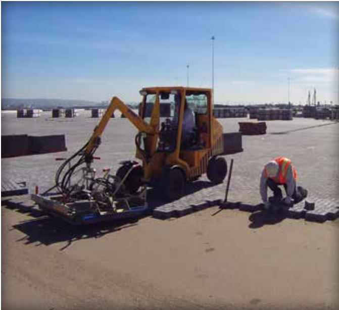
Figure 15. Spacing of cubes at the laying face is determined by how much area will be covered by each, as well as by the clearance required by the machine clamp. Orientation of the cubes follows the direction of paving.
