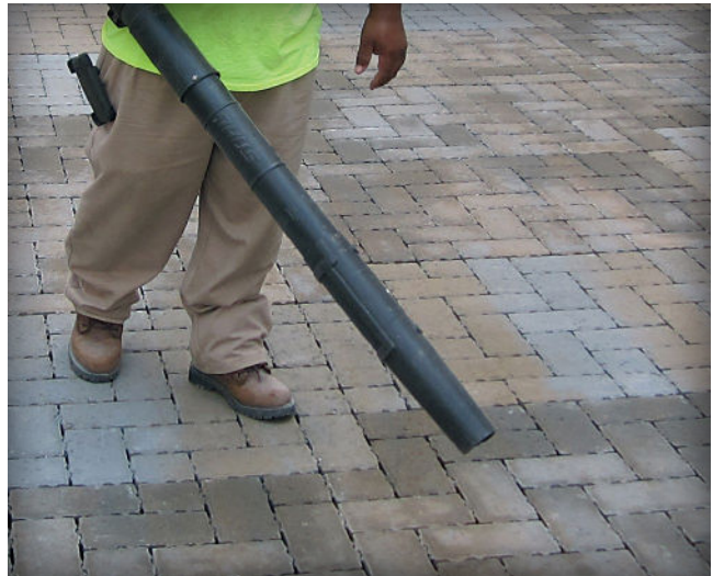
Figure 15. Blowing debris to curbs or gutters for removal and disposal.
