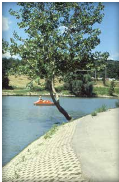
Figure 4. Lakeside stabilization
