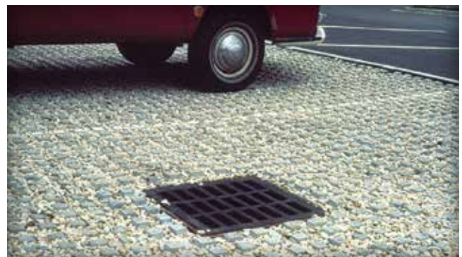
Figure 16. Concrete grids with aggregate in the openings
