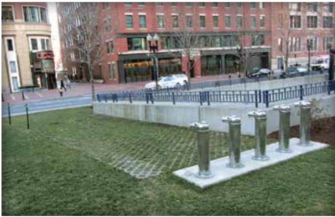
Figure 7. Emergency access lane for fire trucks
