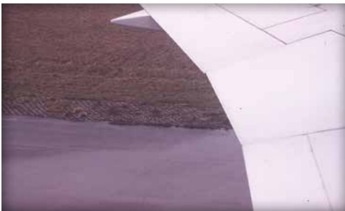
Figure 11. Airfield taxiway shoulder
