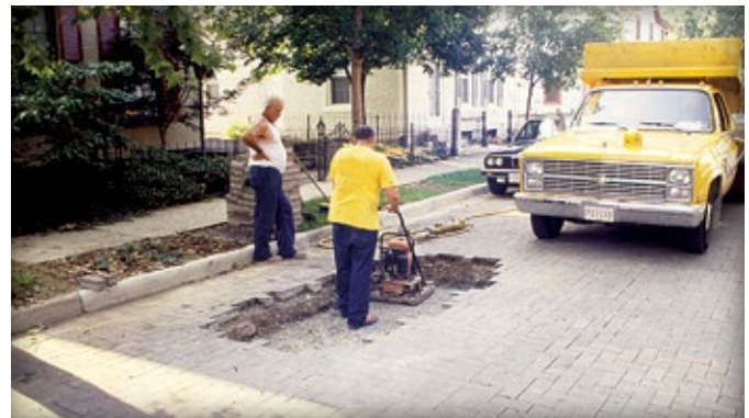
Figure 3. Compaction of the base
