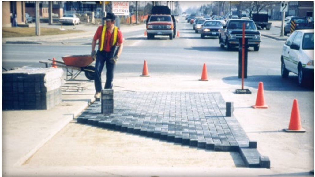
Figure 12. Pavers are laid in a 90 degree herringbone pattern between the border courses.
