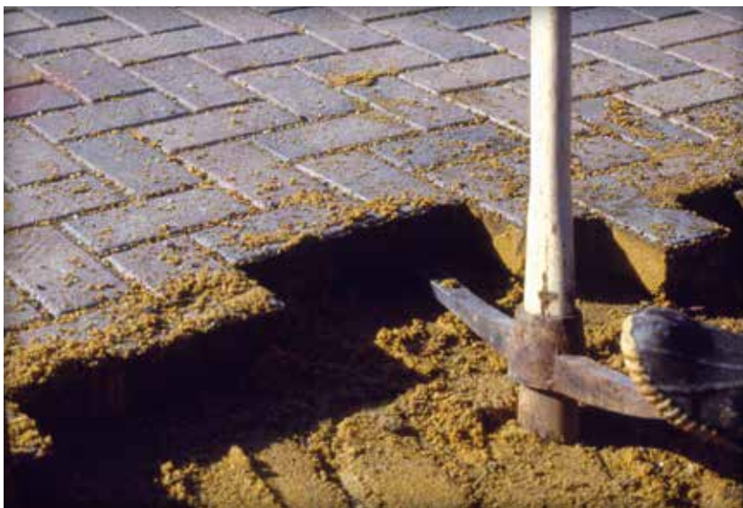
Figure 6. Prying out the remaining pavers
