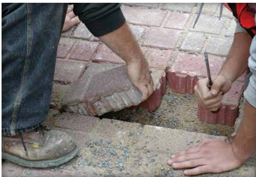
Figure 7. Pulling out a paver by the short end provides greater leverage and makes extraction easier.
