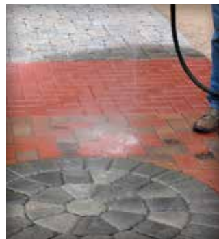
Figure 7. Dry-applied joint sand with a stabilizer is wetted in order to activate it and stiffen the sand. Once the joints dry, they are stabilized.
