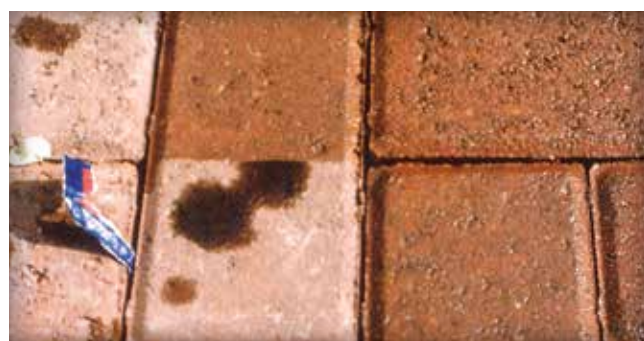
Figure 9. Sealers resist stains which makes them ideal for high use areas where they might occur.
