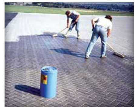
Figure 10. Urethane is applied with squeegees to stabilize joint sand between pavers on aircraft pavement.
