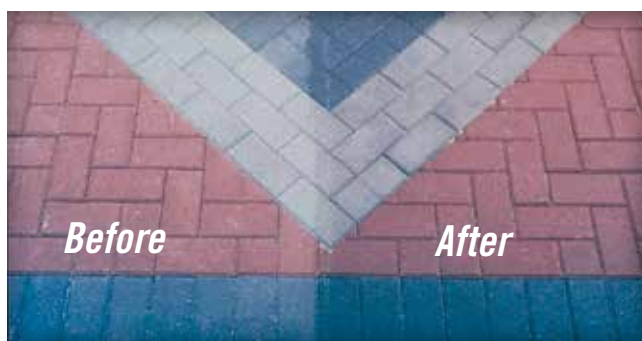
Figure 8. Before and after application of an acrylic sealer shows how it deepens the appearance of concrete pavers.
