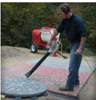
Figure 6. Whether using liquid or dry joint stabilization materials, the surface of the pavers should be cleaned with a blower or broom after the joint sand is compacted into the joints.
