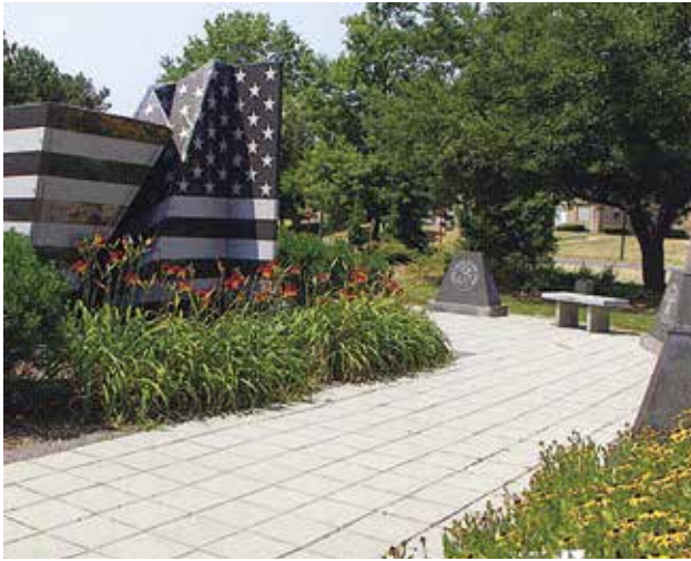
Figure 14. High SR paving slabs
