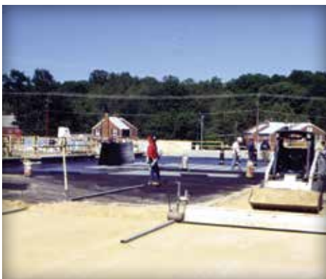
Figure 19. A mechanical screed used to level bedding sand on a roof parking deck project.
