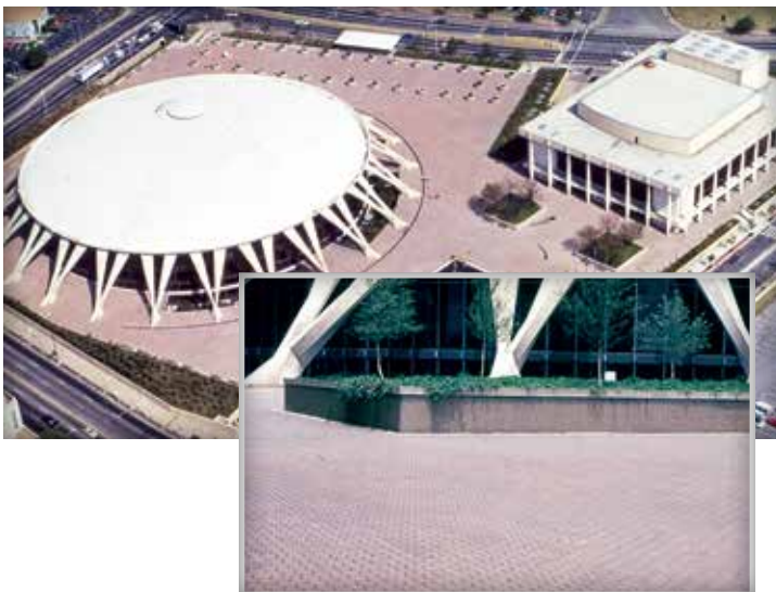
Figure 22. The plaza area around Scope Center in Norfolk, Virginia, (left) and one side of the Alamo Dome (right) in San Antonio, Texas, include roof plaza decks surfaced with concrete pavers.
