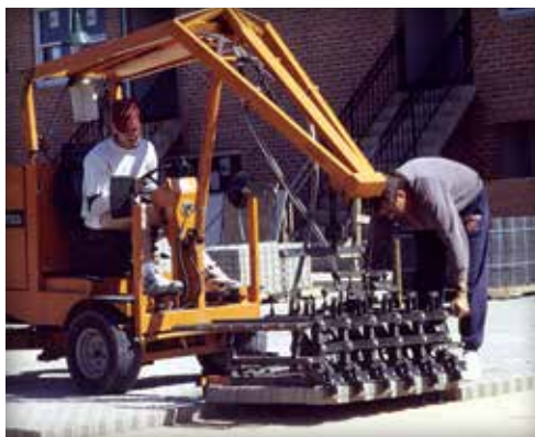
Figure 20. Mechanical equipment used to install concrete pavers on a roof deck.
