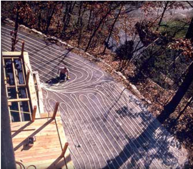
Figure 6. Experienced electrical and plumbing contractors should install snow melting systems.
