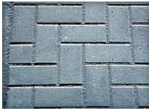
Figure 7. A close-up of the concrete paver surface at the PTI test track.
