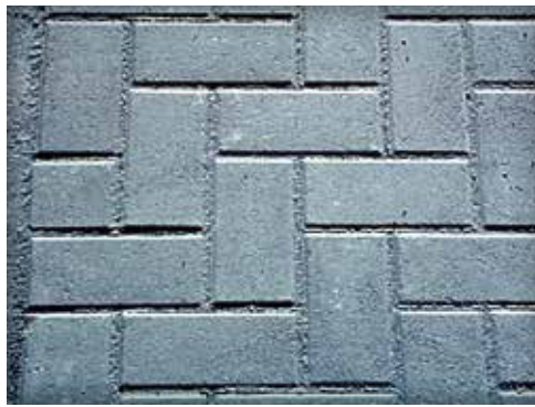
Figure 6. A close-up of the concrete paver surface at the PTI test track.
